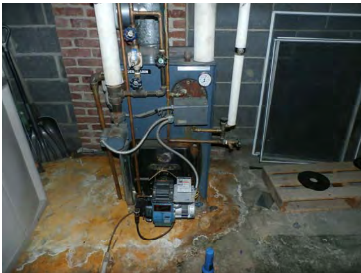
Typical older heating boiler with domestic hot water coil
