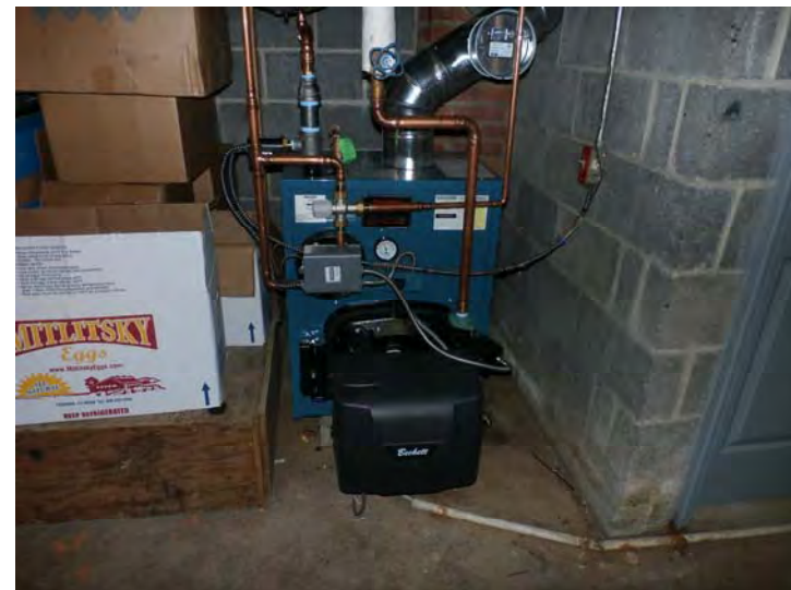
The newly replaced boiler with DHW coil
